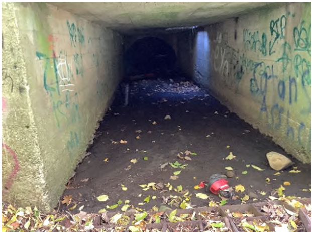
Photo 4: View of the Bank present within Walker Brook culvert.
