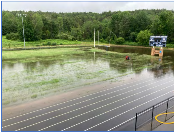
Figure 14. Flooding at the Wahconah Regional High School.
