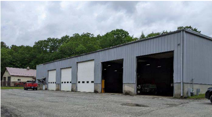
Fig. 2: Front of parking lot and half of the garage are all impervious surface with no stormwater treatment. Infiltration near street may be an option. Source: UNH Stormwater Center
