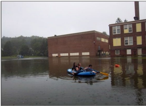
Rafting during flood event at former High School Source: Old Dalton High School Advisory Committee
