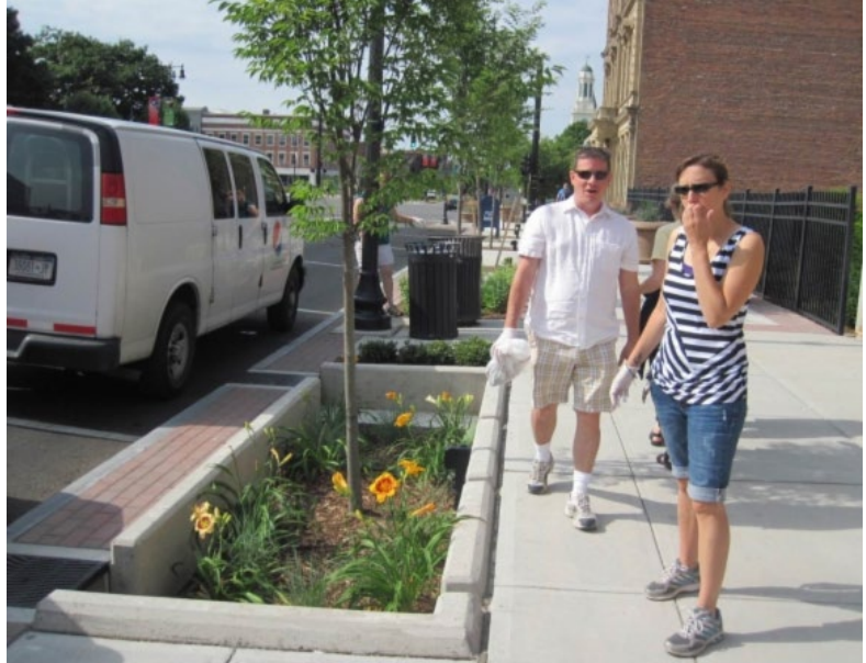
The City of Pittsfield installed 10 rain gardens on North Street by 2014. Source: City of Pittsfield
