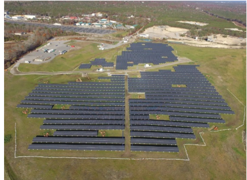
Location: Falmouth, MA Size: 4.0 MW Technology: Ballast on muni landfill
