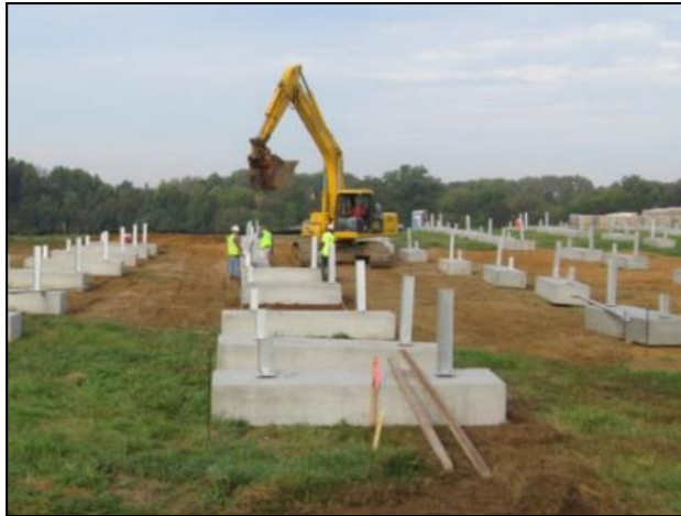
Installation of non-penetrating ballast blocks with Low Ground Pressure Equipment (LGPE)
