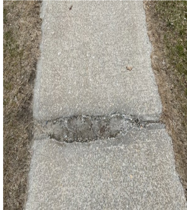
HC Ramp to enter Police Station & Town Hall lacks slip resistant surface and is not ADA compliant; deep grooves in pavement create a danger and obstacle to wheelchair use
