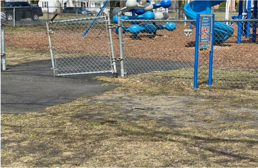
No Safety Surface at playground
