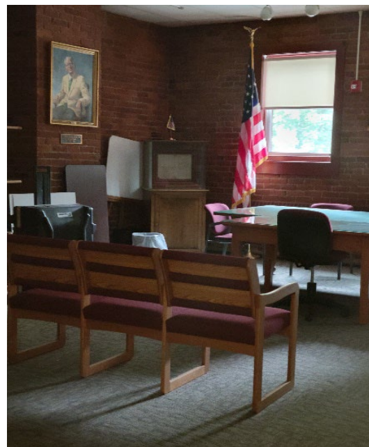
Callahan Meeting Room is minimally accessible, but wheelchairs cannot pivot
