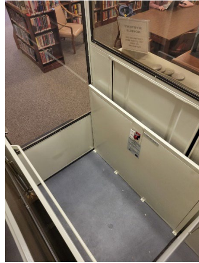
Lift to City Hall & Restrooms
