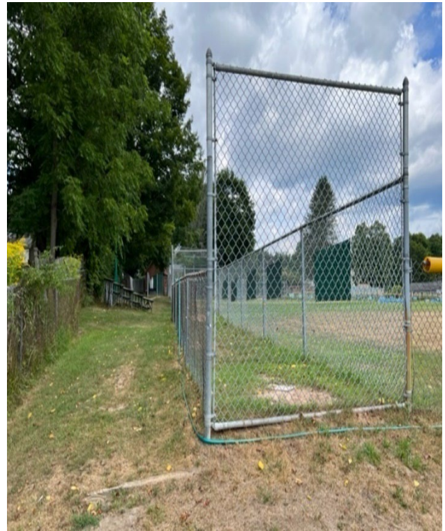
Non-ADA compliant route to the bleachers
