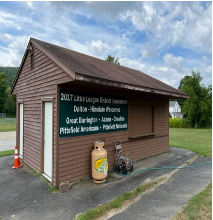
Restroom Entrances lack signage and
