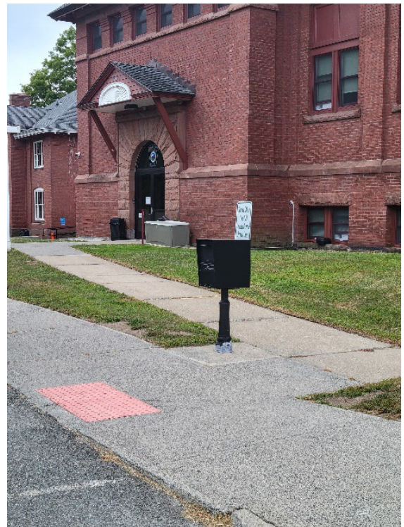
Ramp to Police Station Entrance
