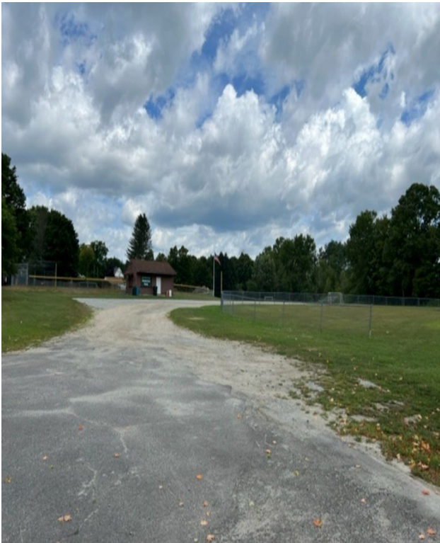
Entrance to Chamberlain Park – no ADA parking
