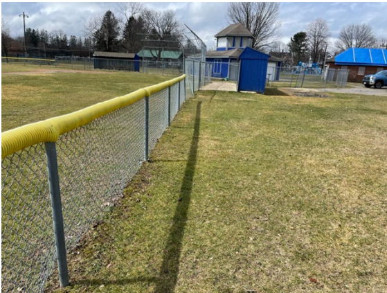
No accessible path to Bleachers
