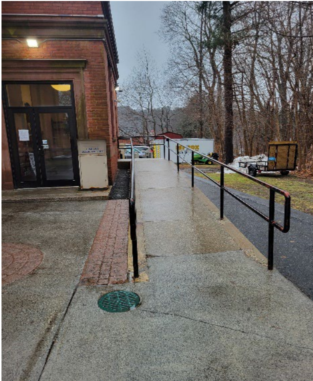
ADA Ramp to Library
