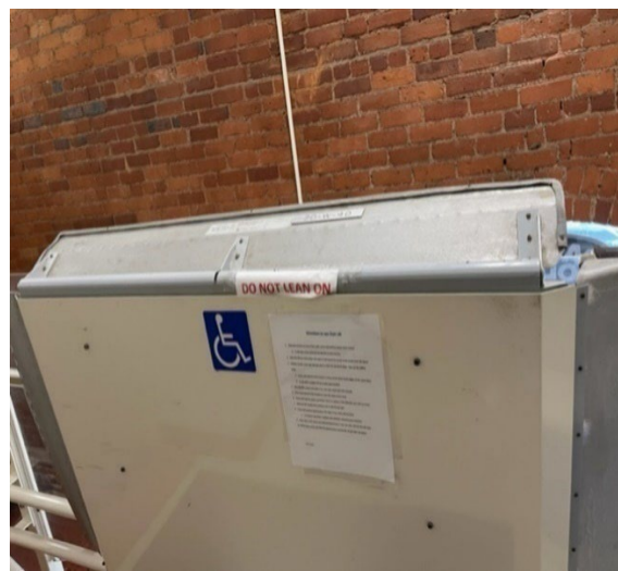
Existing chair lift does not allow independent use; and accesses Town Hall main floor but not Police Station
