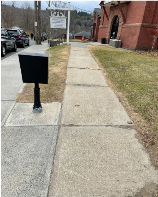
HC Ramp to enter Police Station & Town Hall lacks slip resistant surface and is not ADA compliant; deep grooves in pavement create a danger and obstacle to wheelchair use
