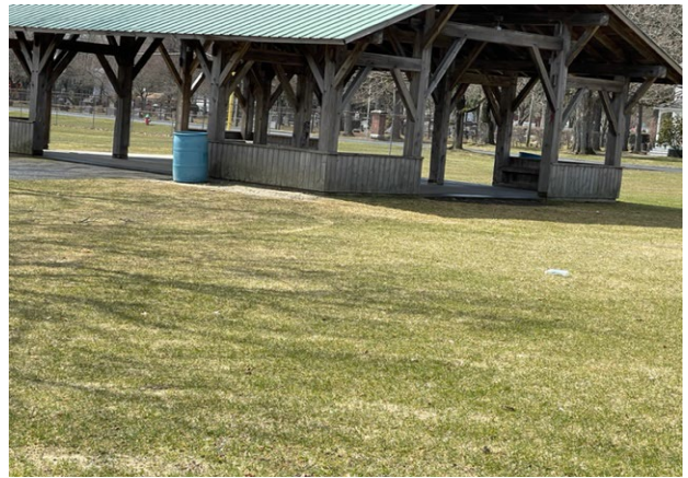
No accessible path to Pavilion
