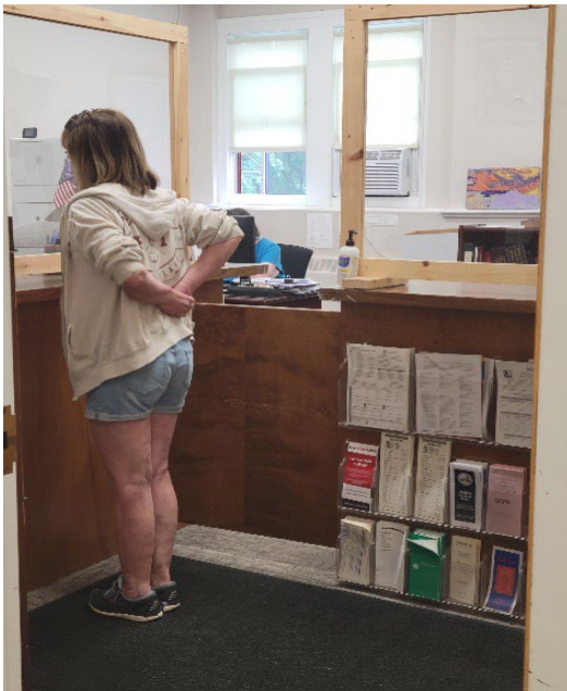
Service counters in offices do not meet ADA requirements for wheel-chair use
