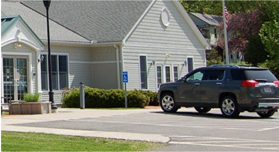
Senior Center Handicap Parking and signage
