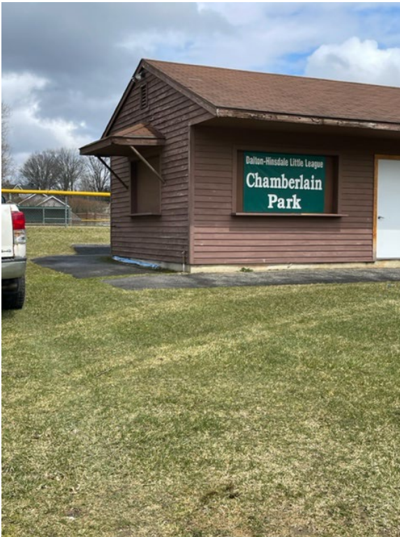
Concession Stand - no accessible route accessibility
