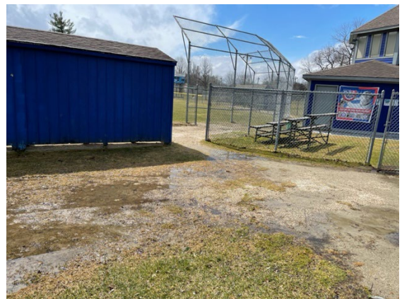
No ADA Parking or ADA path to Bleachers
