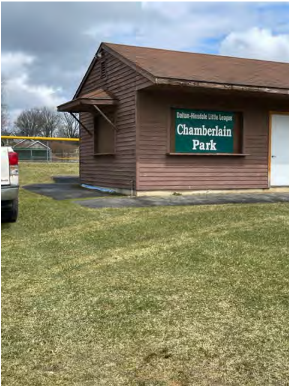
Concession Stand - no accessible route accessibility
