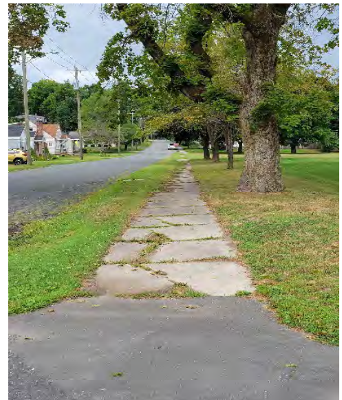
First St – looking west
