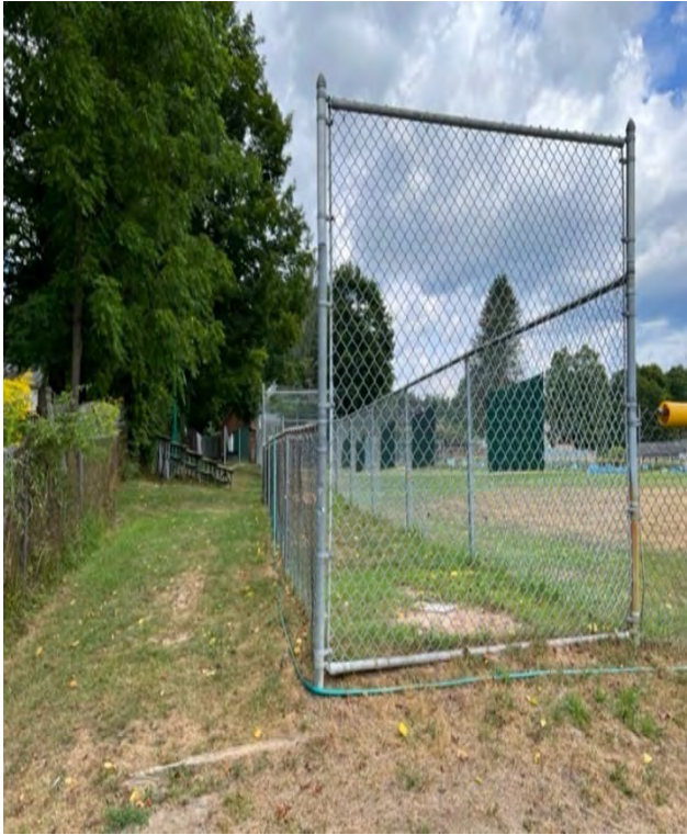
Non-ADA compliant route to the bleachers
