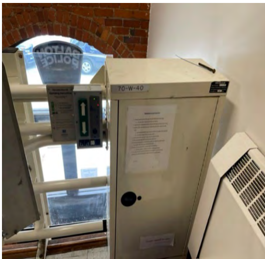
Existing chair lift does not allow independent use; and accesses Town Hall main floor but not Police Station
