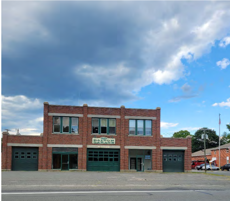
Garage – Main Street
