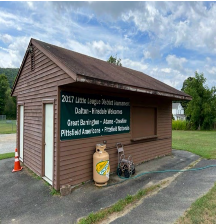
Restroom Entrances lack signage and
