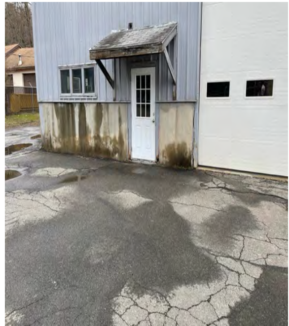
No signage or ADA parking at
