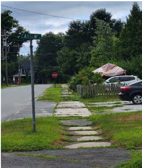
Looking down First Street / Carson
