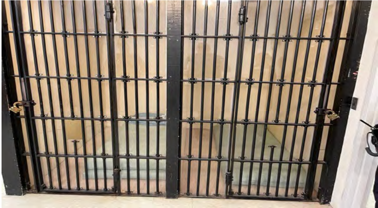
Holding Cell at the Police Station
