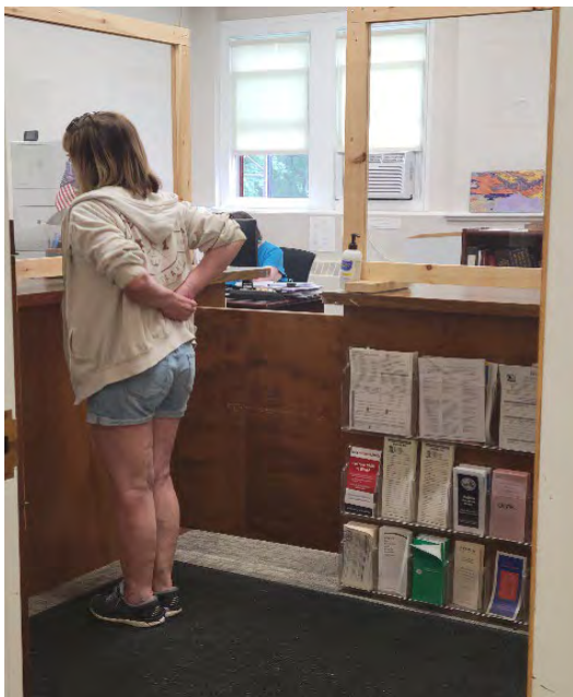
Service counters in offices do not meet minimally ADA requirements for wheel-chair use pivot
