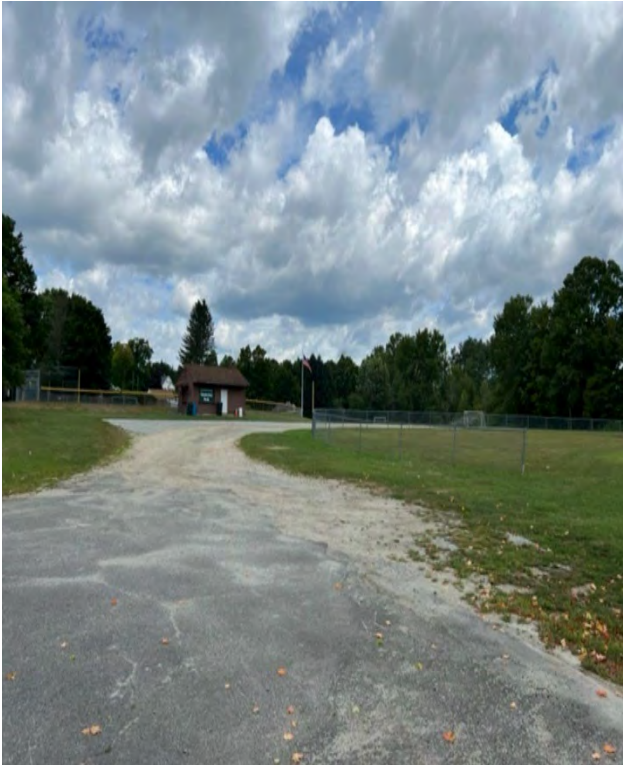
Entrance to Chamberlain Park – no ADA parking
