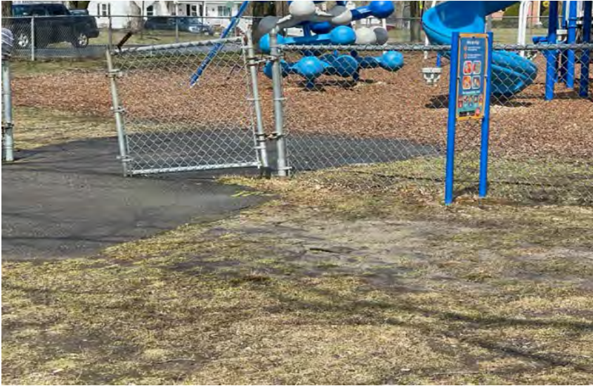
No Safety Surface at playground
