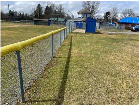
No accessible path to Bleachers Bleachers
