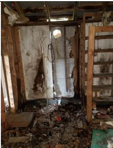
Photo 5: View of possible furnace room in the garage. The hole in the wall near the ceiling appeared to connect to an exterior cinder block chimney.
